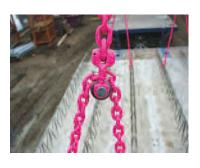
Ensures even load distribution by means of a compensating pulley with a VVGSCH-8. There is neither overload nor deformation of the concrete element.
