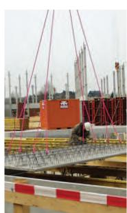
VIP-**Balancing** assembly "VIPoctopus" for concrete elements
